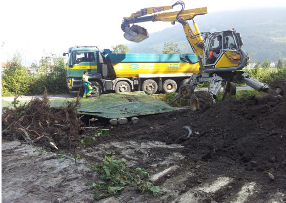
Abtransport belastetes Material
